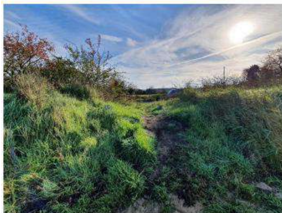
Remblai routier – ISL 2024
